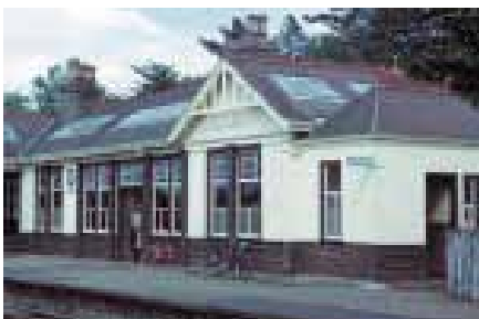
New railway station.
